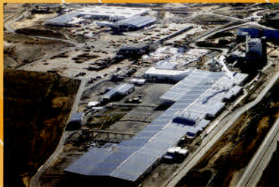
Aerial view of our new state-of-the-art Nueva Aldea plywood plant, north of Concepcion, Chile
